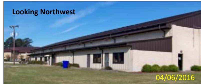
2016 South (Front) Exterior
